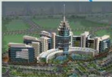
DSO's impressive headquarters — open from April 2007.
