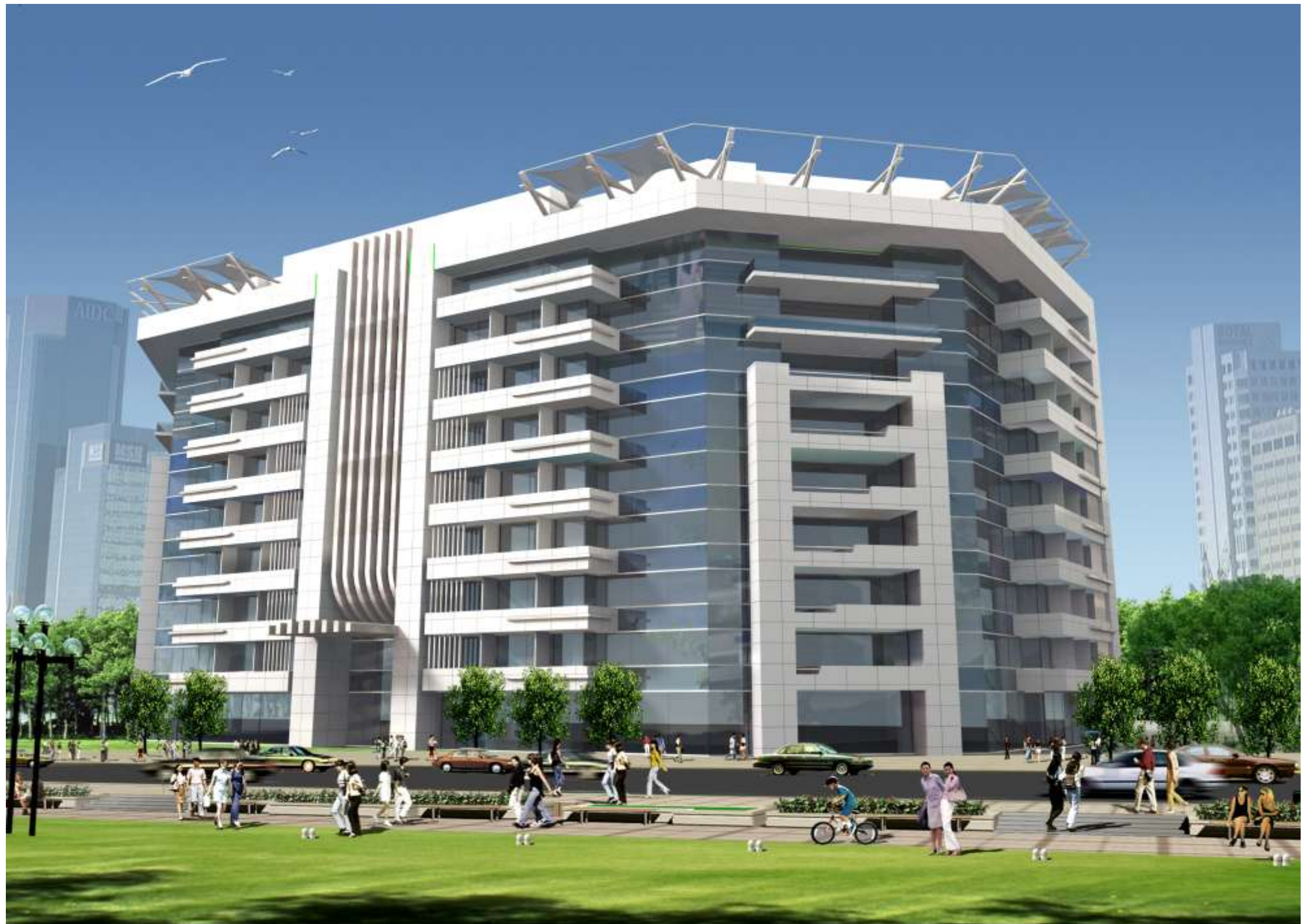
Silicon Height Residential Building at Dubai Silicon Oasis
